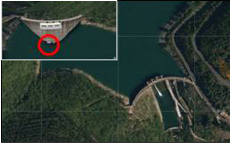
The aerial photo shows the entire dam structure and the targeted inspection area.
